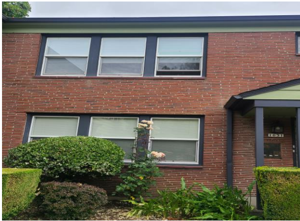
Brick & Mortar-Clean & Seal
