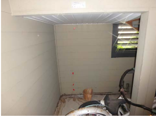
2.2.34. Overview of IO 9, the interior wall to IO 14
