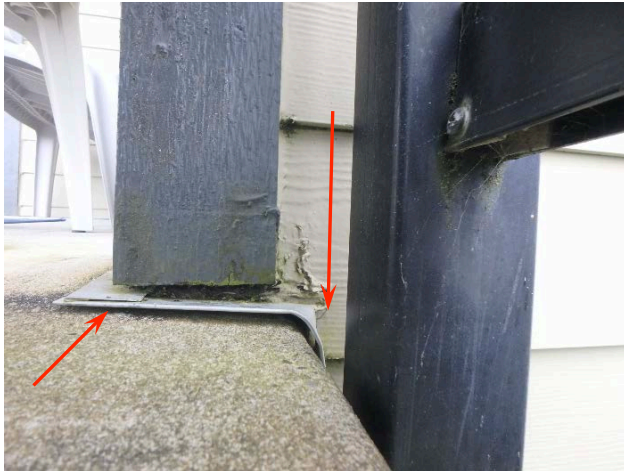
2.4.12. Omitted or discontinuous flashing "diverter" at deck-to-wall flashing termination
