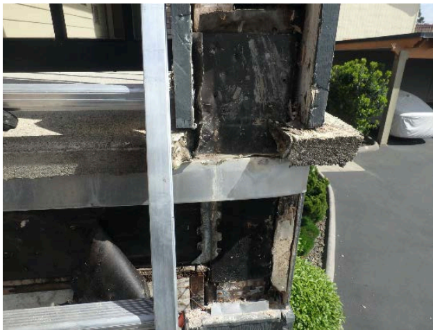
2.3.10. Overview of saturated beams below the walkway assembly
