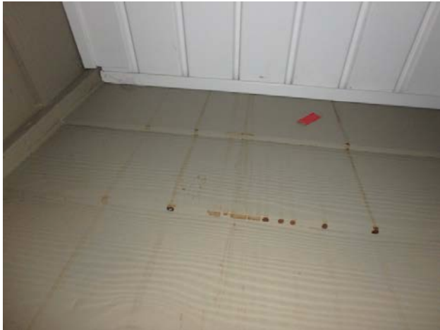
2.2.35. Moisture staining emanating from within wall assembly
