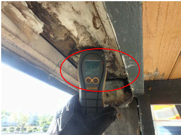
2.3.9. Greater than 19% MC in front walkway structural beam
