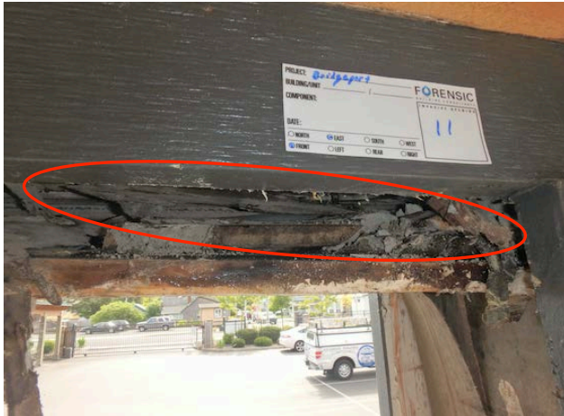
2.3.8. Moisture-deteriorated gypsum sheathing below structural beam assembly
