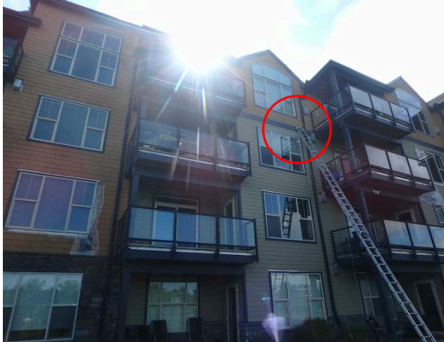
2.1.14. Overview of IO 15 at third floor window head
