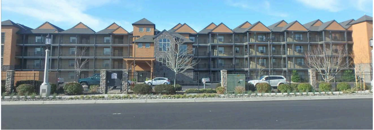
1.1.1. Overview of front/east elevation
