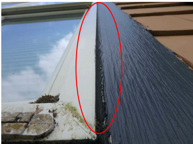
2.1.15. Overview of fenestration condition on the fourth floor above IO 15
